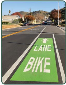
Colored Bicycle Lane Markings
